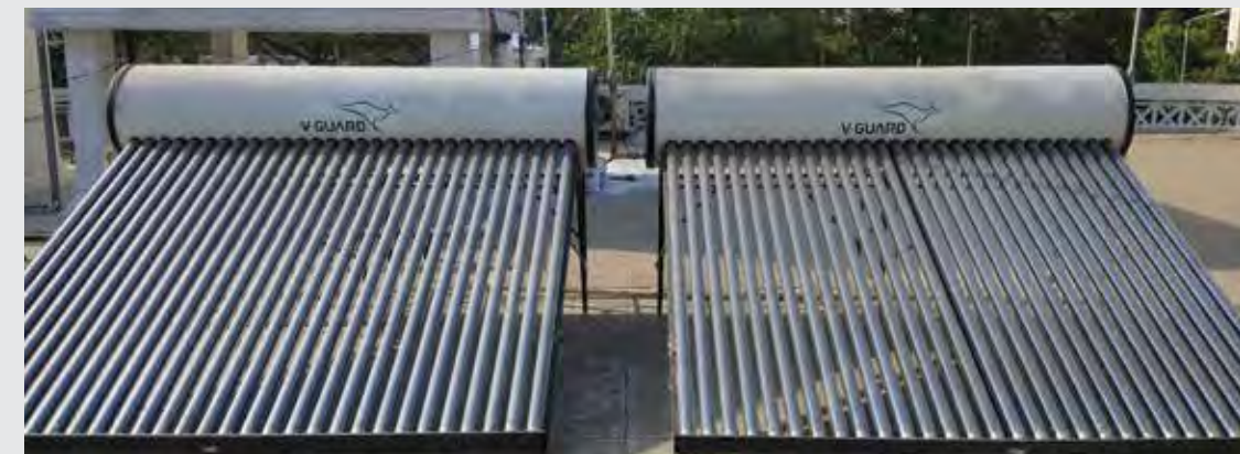
Solar Panels installed at Mahape
